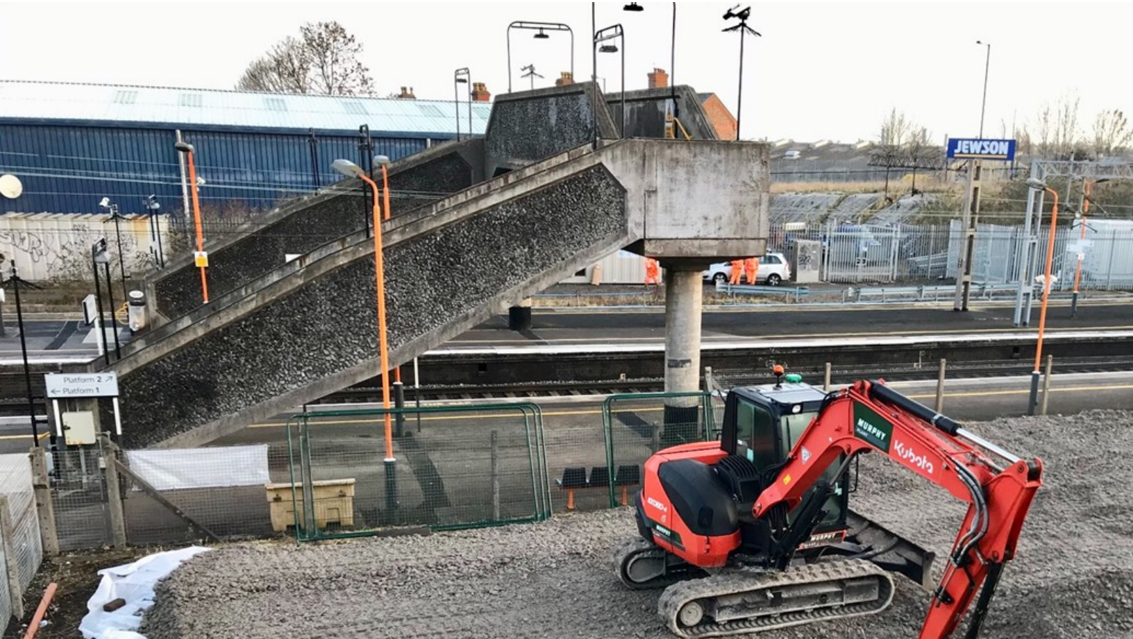
Ground work taking place at Stechford station
