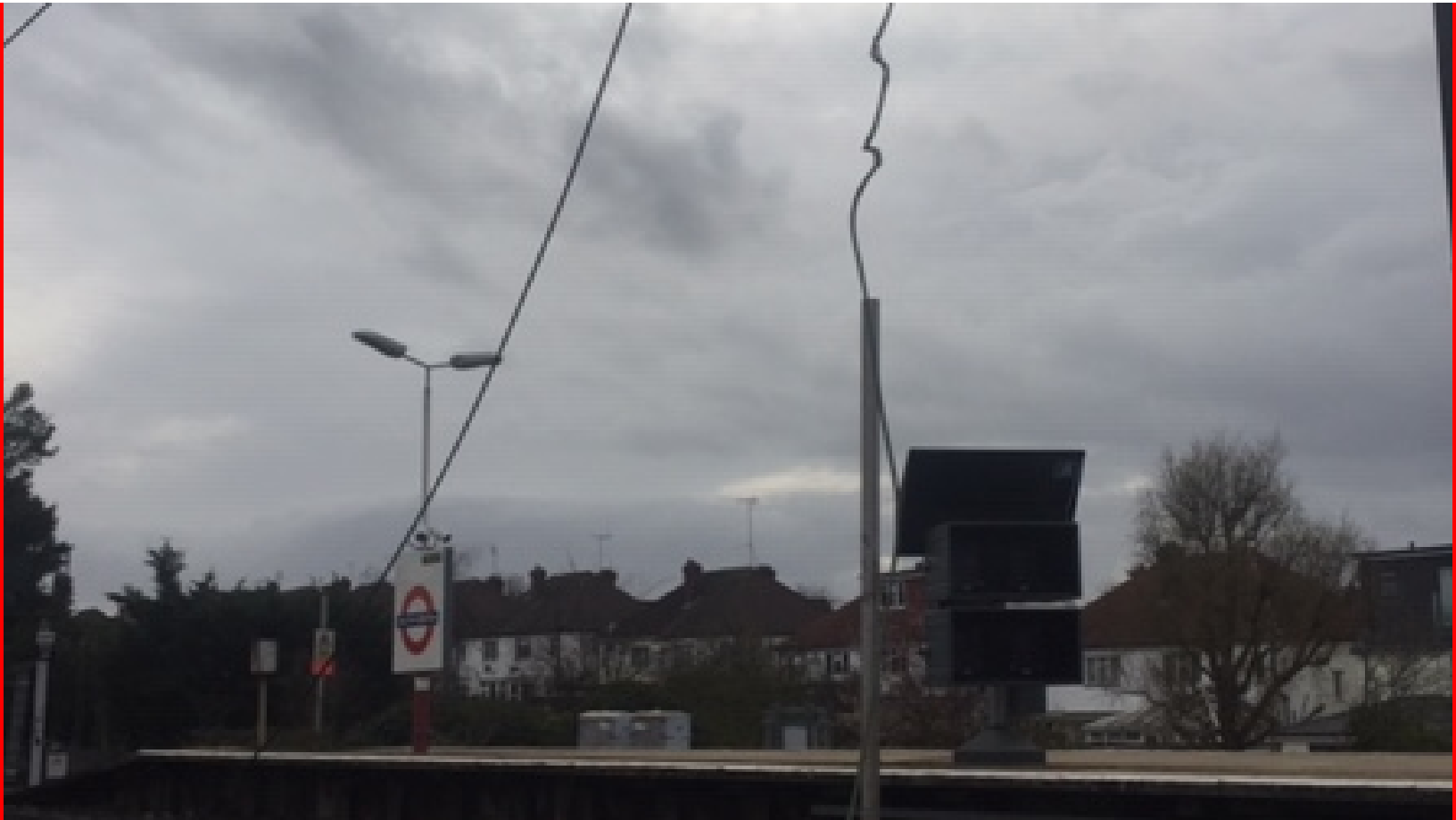
Damage to overhead power lines outside Euston
