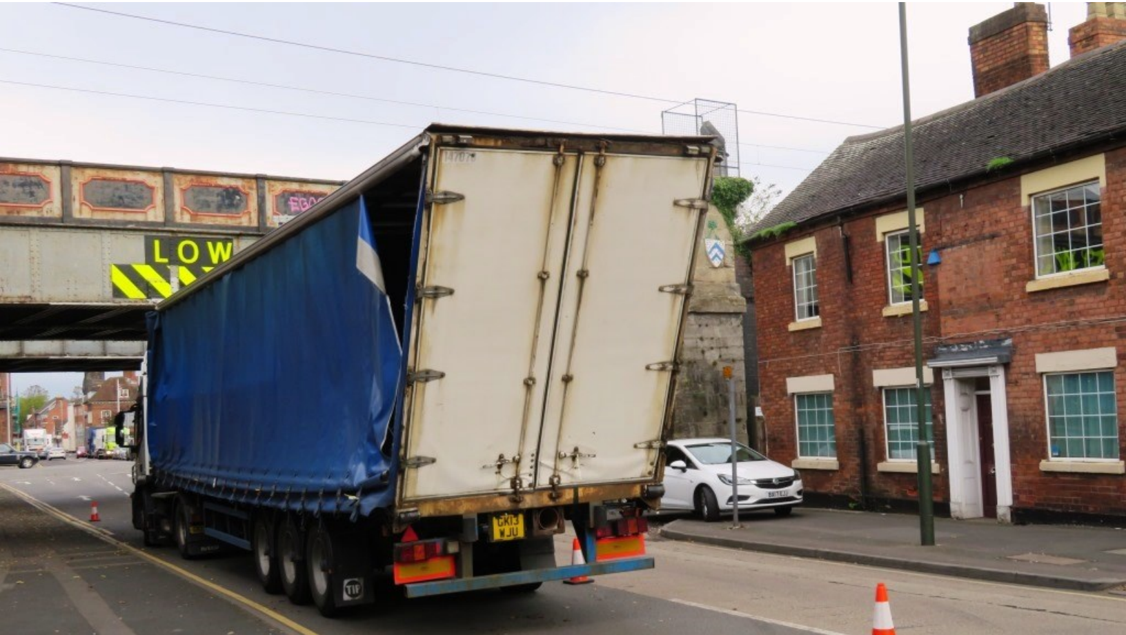
The St John's Street bridge in Lichfield
